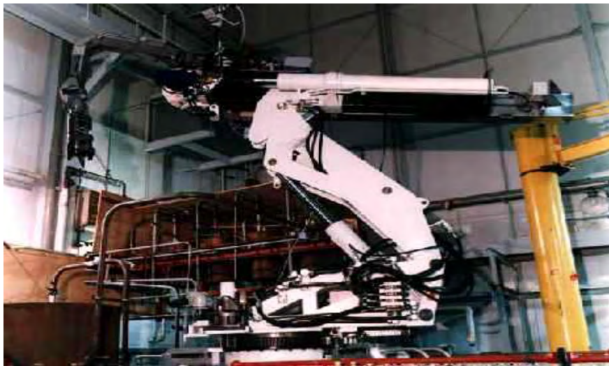
Fig. 2. Remote Decommissioning Handling
