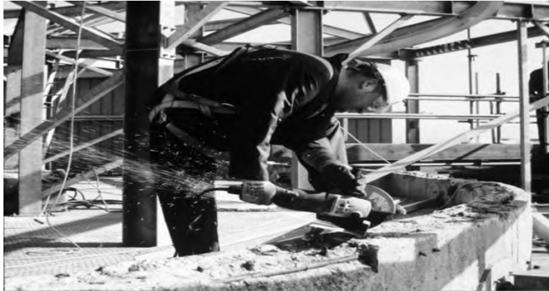
Fig. 1. Manual Decommissioning Technique
